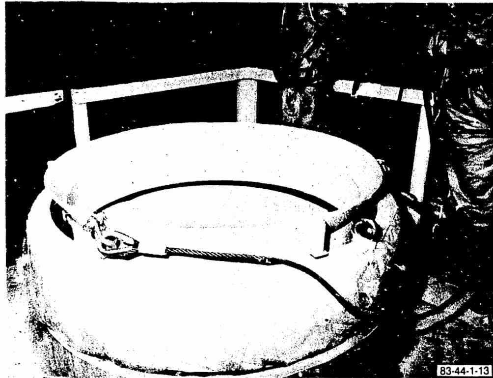
Figure C-6. Photograph of the liner interface collar placed in an HIC.
